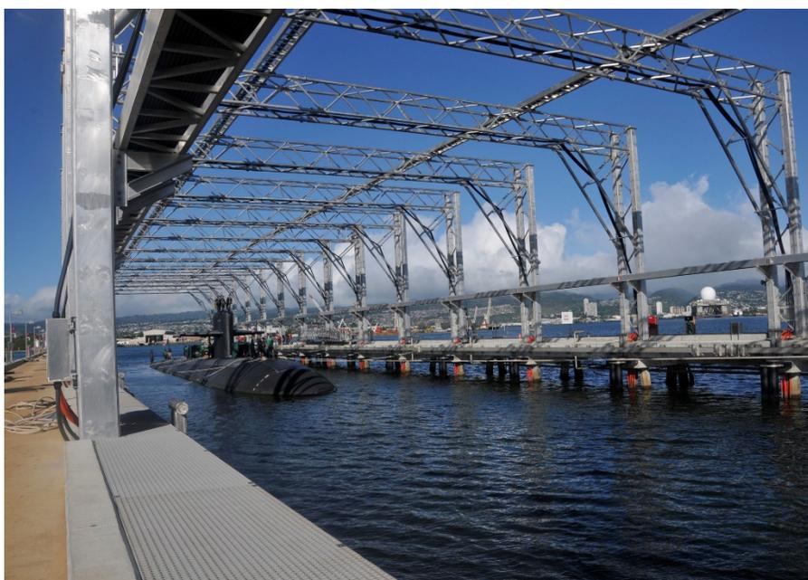
De-perming doesn't eliminate the magnetic field but it minimizes it, makes it constant and predictable. For the sake of crew safety, navigation, and performance, controlling the magnetic field prevents the United States from having a Magnetic Navy.
